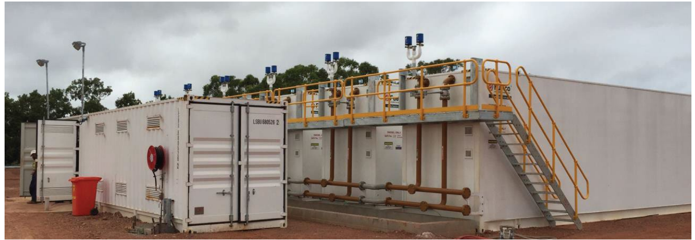
METRO MINING - 600,000L diesel fuel farm. 1x Adblue tank at remote site mine in North Queensland
