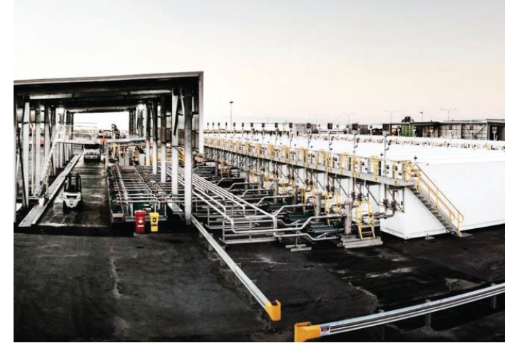
CASTROL BP - 43 x Logitank LSB110 self bunded tanks, totalling 4.7 million litres of storage for 16 lubricant products
