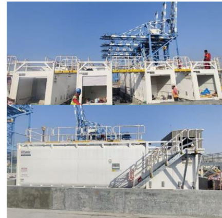
Fuel Depot for a Port in UAE 4xLTKB 47 – 2 hours Fire rated tank. Capacity – 47,000L GFL per tank
