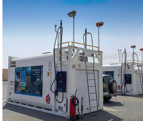
UL 2085 FIRE RATED TANKS FOR FUEL STATION, OMAN
